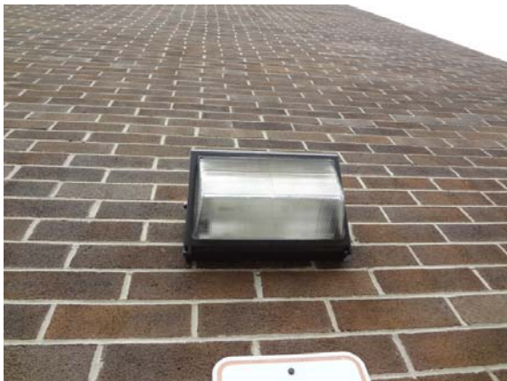
Photo #21: Brick veneer recently repointed and coated, surface mounted lighting
