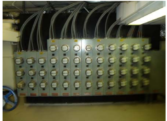
Photo #40: Electric meters in boiler room
