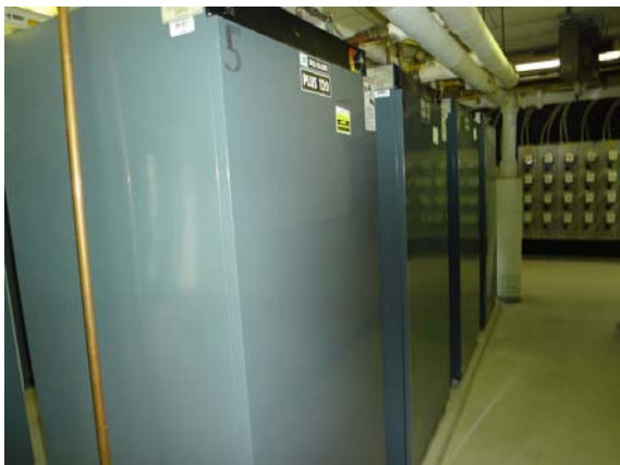
Photo #35: Water heaters connected to domestic boilers
