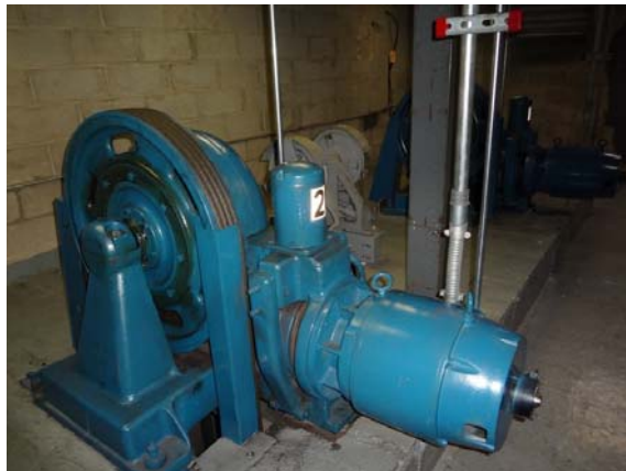
Photo #43: Elevator machinery
