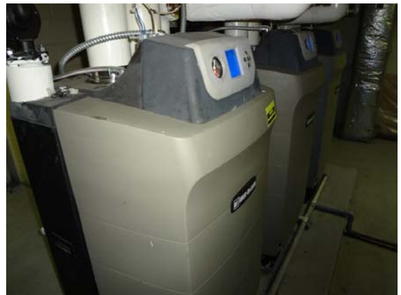
Photo #34: Domestic water boilers
