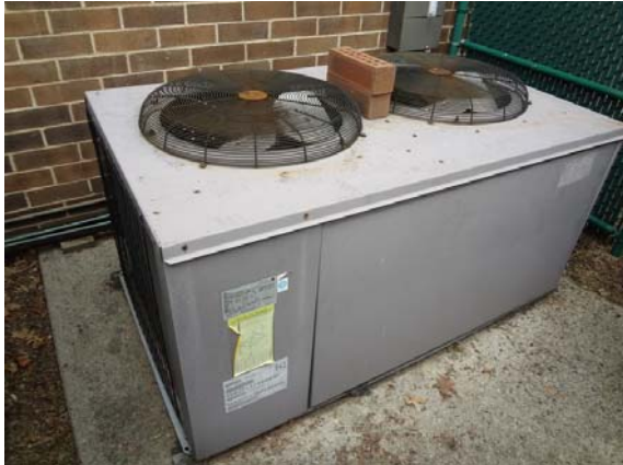
Photo #37: Smaller condenser for community room air handler
