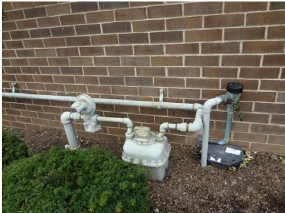
Photo #39: Gas meter assembly
