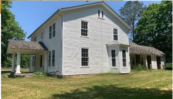
Hammond House rear section, 1818 front section 1836
