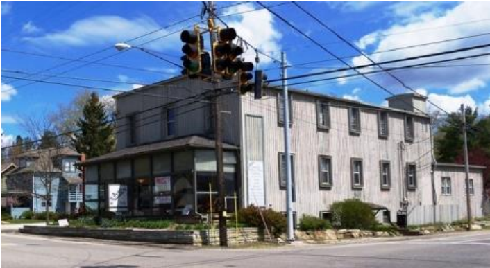
Garth Andrew’s Interior Design Store 1969 N. Cleveland-Massillon Rd.
