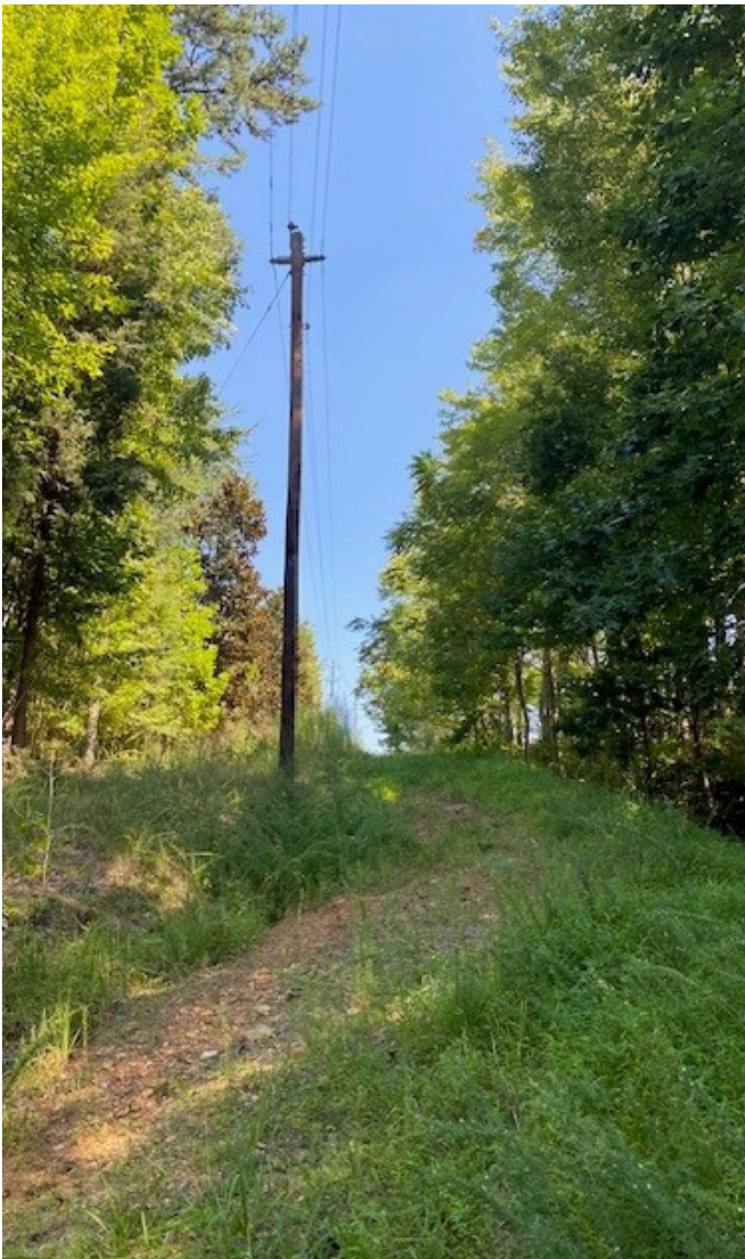
Overhead power lines and steep topography near Vision Dr
