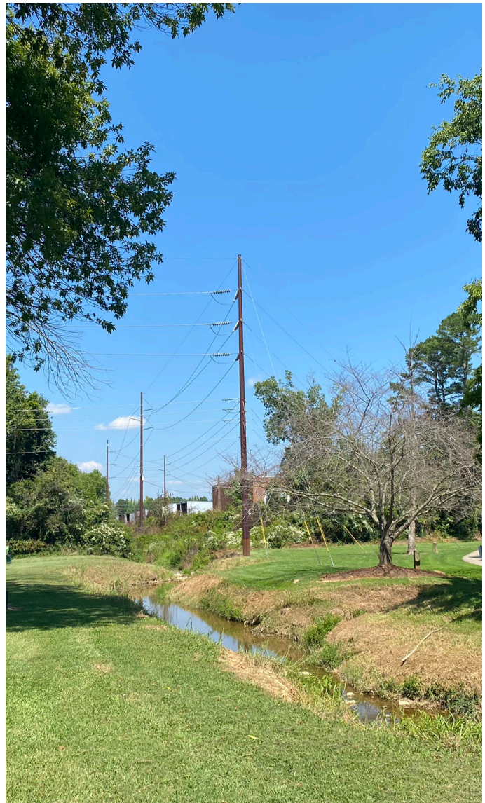
Transmission lines along Hasketts Creek
