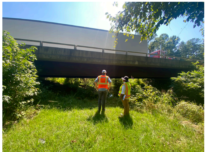
W Central Ave bridge at Hasketts Creek
