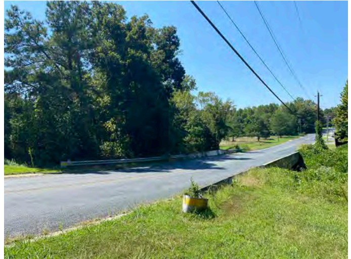
W Bailey St bridge over Hasketts Creek
