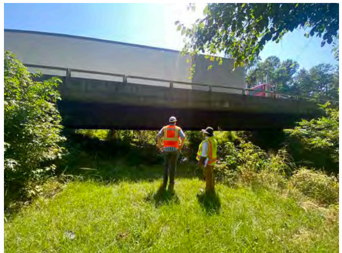
W Central Ave bridge at Hasketts Creek
