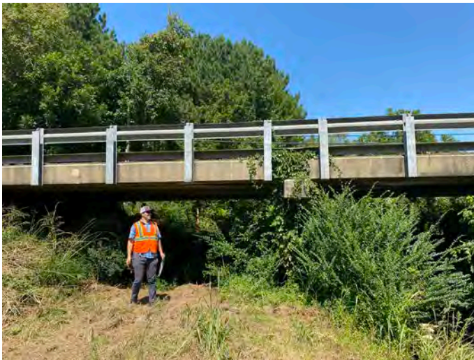
W Balfour Ave bridge at Hasketts Creek
