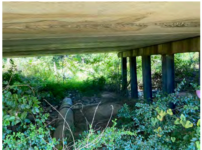
Sewer line under W Balfour Ave bridge
