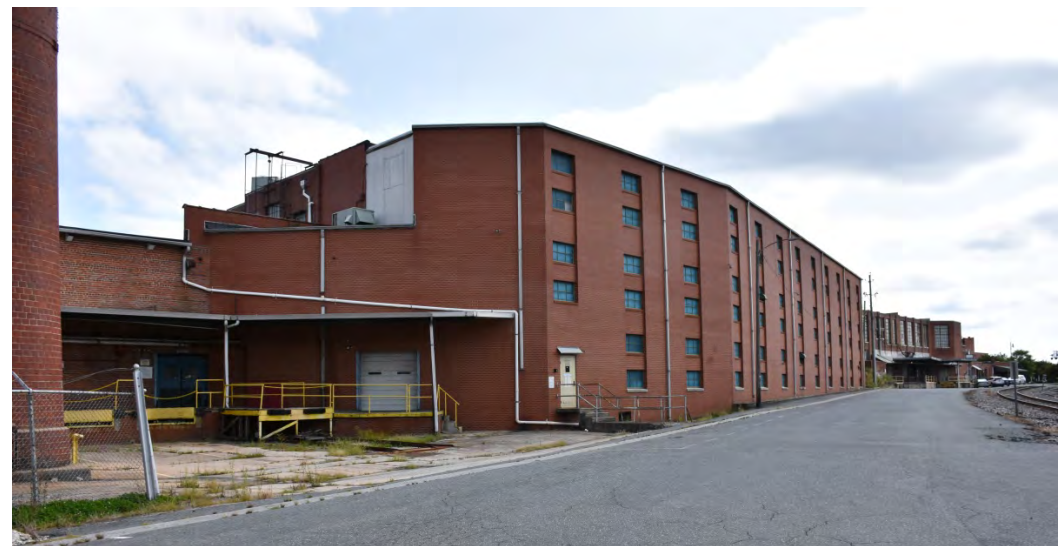
West elevation, 1929 additions at foreground (top), 1928 and 1929 additions (center) and 1962 addition, northwest oblique (bottom)
