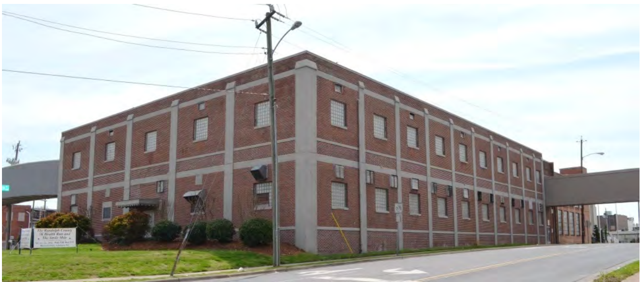
1937 addition, east elevation (top), northeast oblique (center), northwest oblique (bottom, April 11, 2014)
