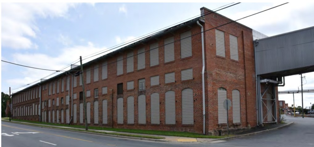
Looking north (top), 1910s addition with 1947 second story south elevation (center) and northwest oblique (bottom)
