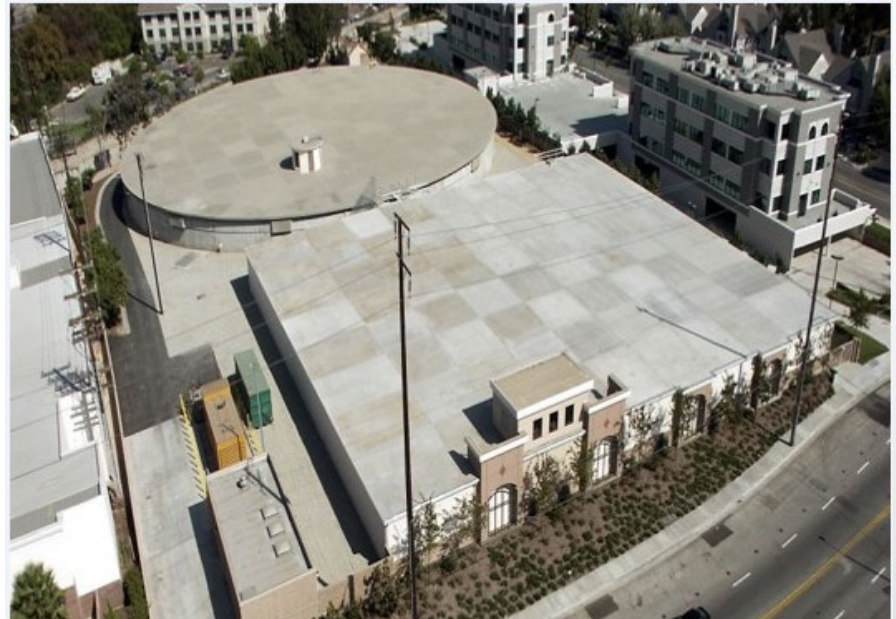
Potable water reservoir
