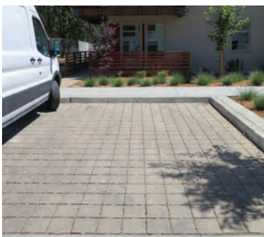
Figure 4.13 DO install permeable paving whenever possible.
