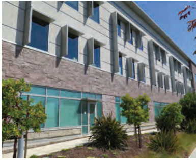
Figure 4.2 DO use a variety of materials and textures to articulate building façades.
