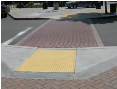
Figure 4.8 DO install patterned or colored paving to alert drivers to pedestrian paths that cross driveways or parking areas.
