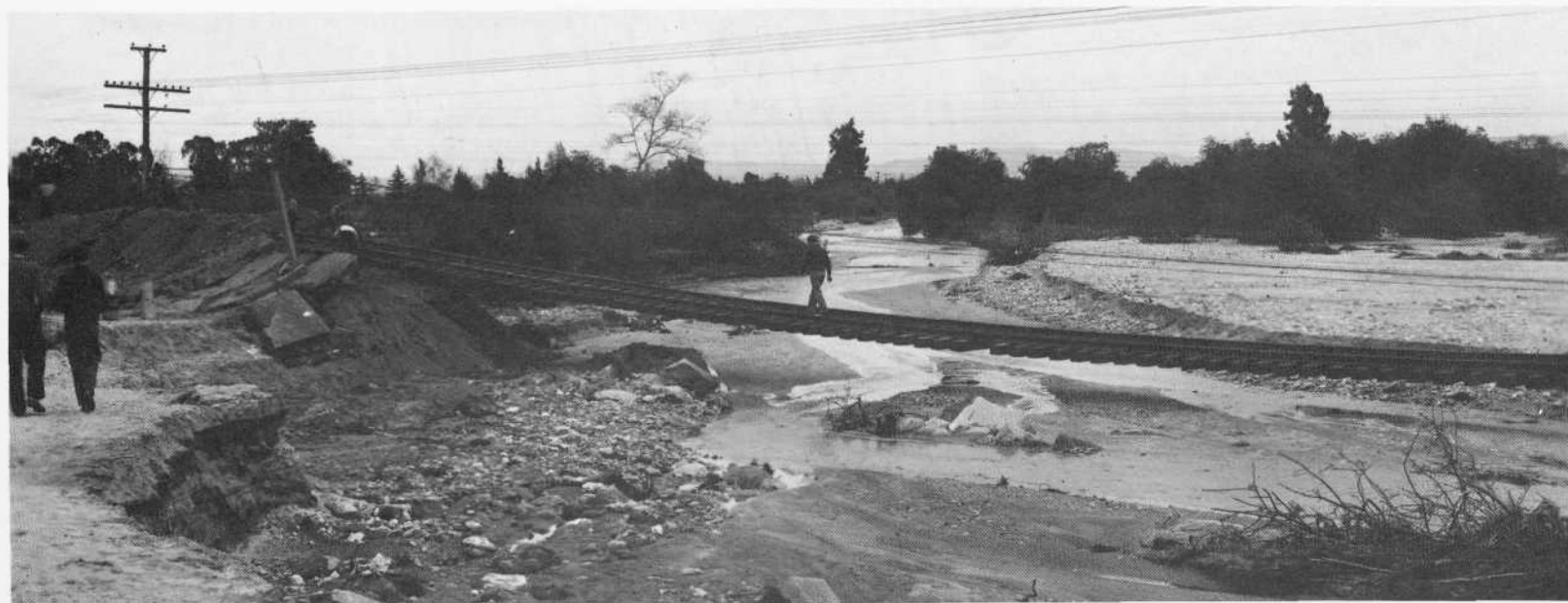
Big Santa Anita Canyon Wash following torrential rains, March 1938. This photo, taken from Huntington Dr. looking north, shows about 300 feet of Santa Fe tracks left in midair. — LOS ANGELES COUNTY FLOOD CONTROL DISTRICT
