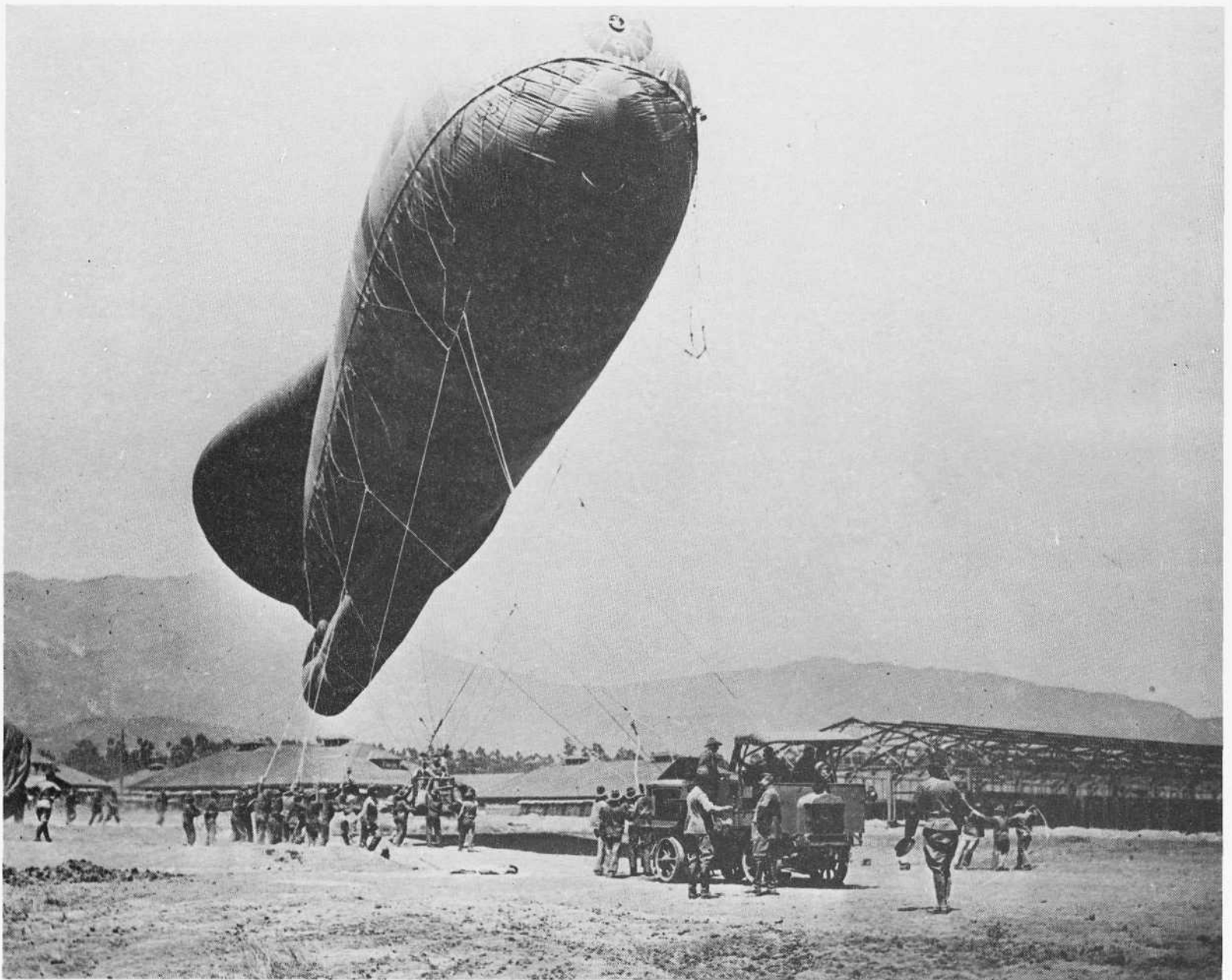
Ross Field personnel preparing to launch observers, 1918. Both Alice Wood and Earl Kramer, early residents, recall seeing one of these baskets fall to the ground in a severe wind storm. (RIGHT) Close view of one of the large captive balloons, so designated because they were anchored to heavy military vehicles, as shown here, circa 1917. — GRADY PARDUE
