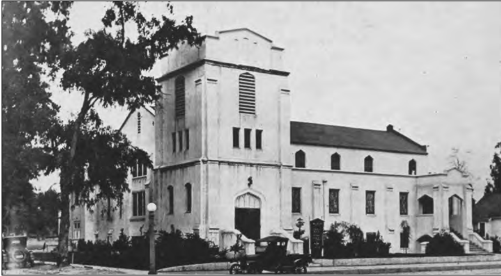
The Community Church, on the northeast corner of Santa Anita Avenue and Huntington Drive, was later cut in half and moved to the corner of First Avenue and Alice Street, circa 1920s.
