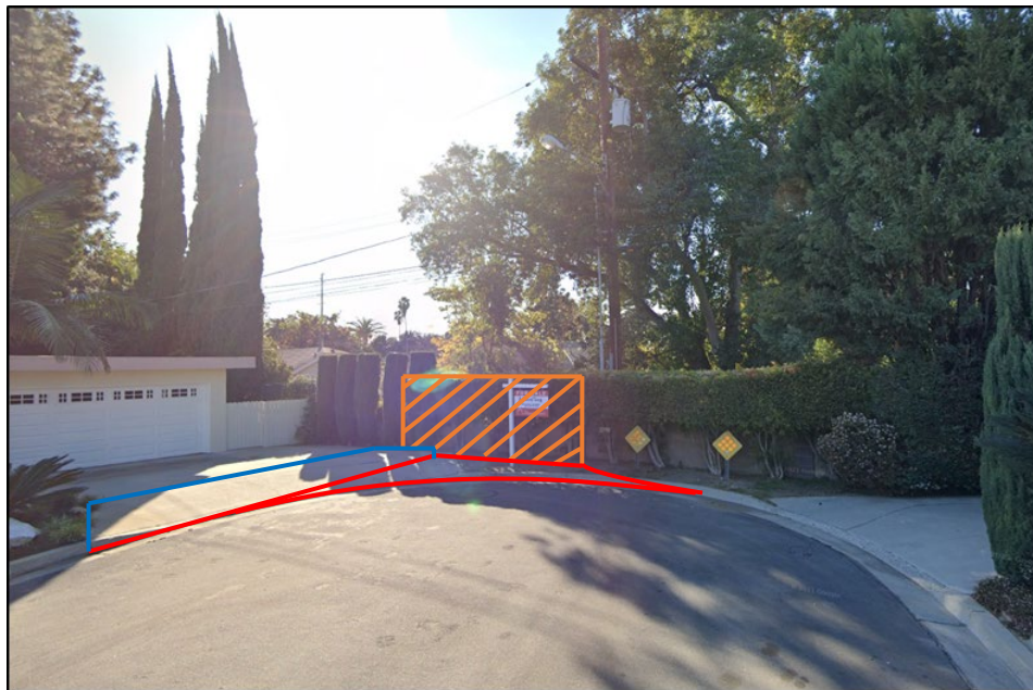
— Street Area to be Paved — New Driveway Apron — Wall in the Right-of-way to be Removed
