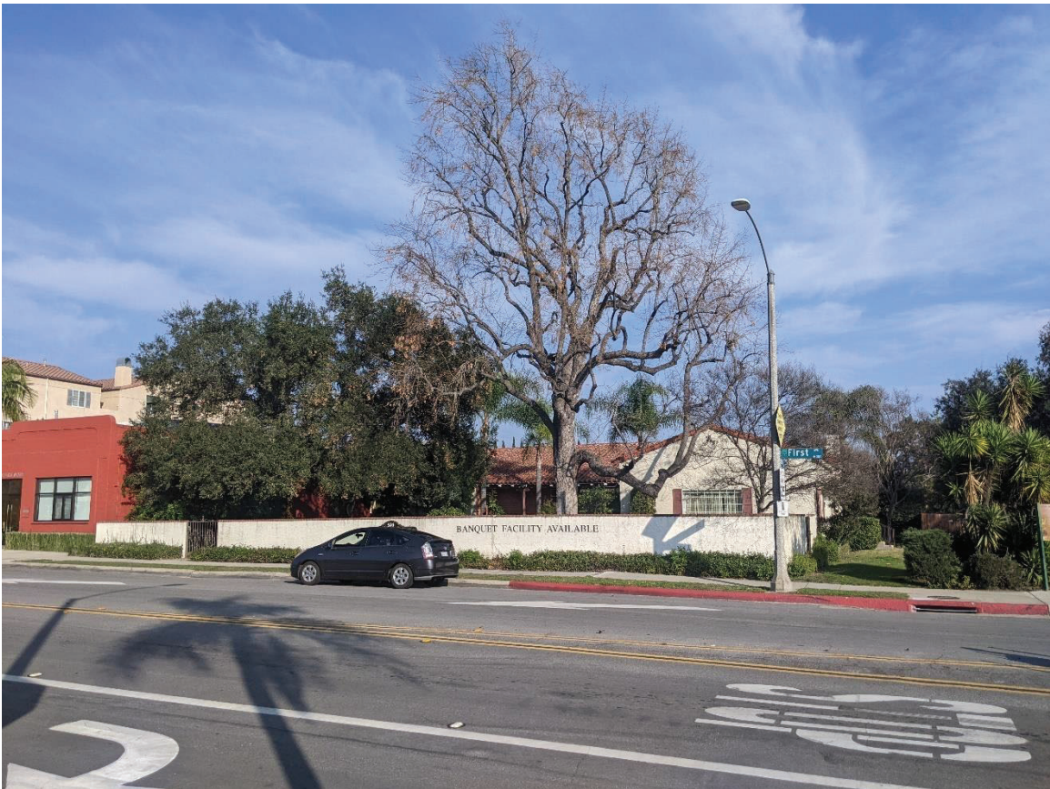
Figure 4 Looking east toward the front facade of the Arcadia Woman's Club building
