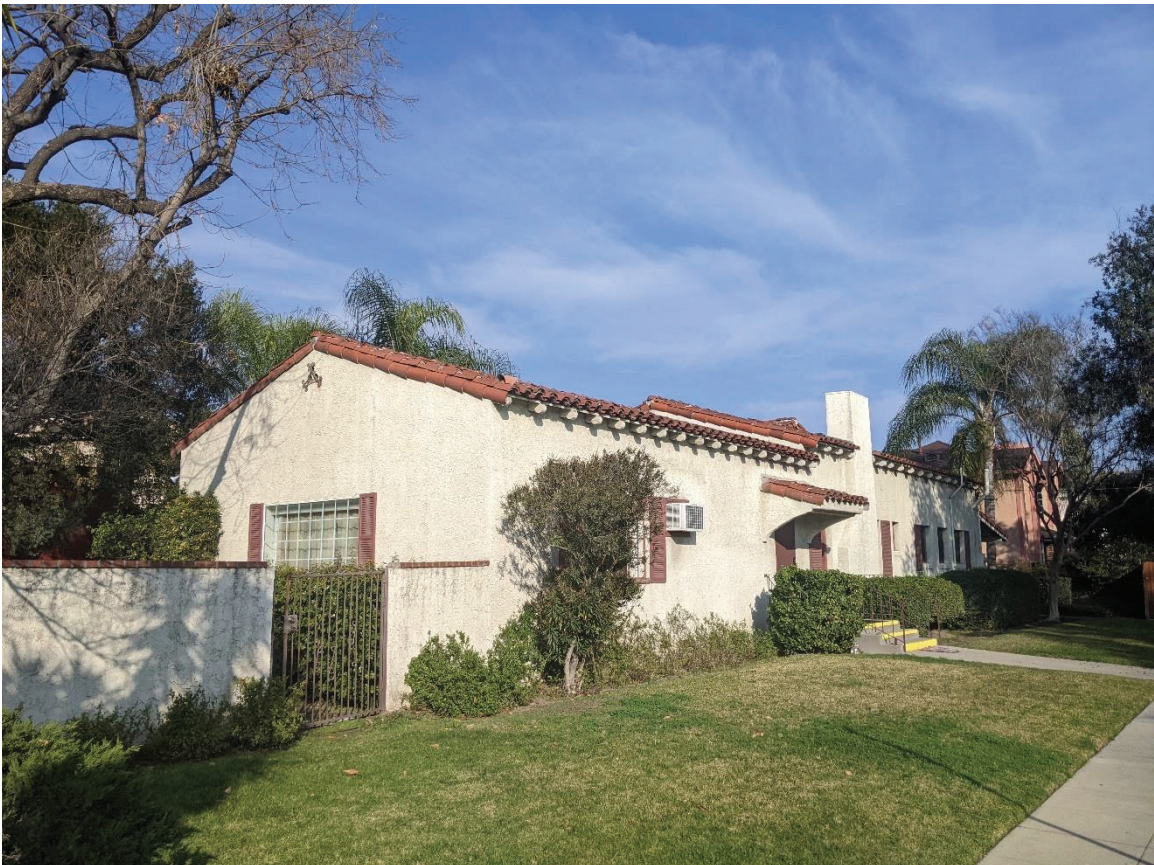
Figure 8 Looking toward the Arcadia Woman's Club building from the corner of Diamond Street and S. 1st Ave.
