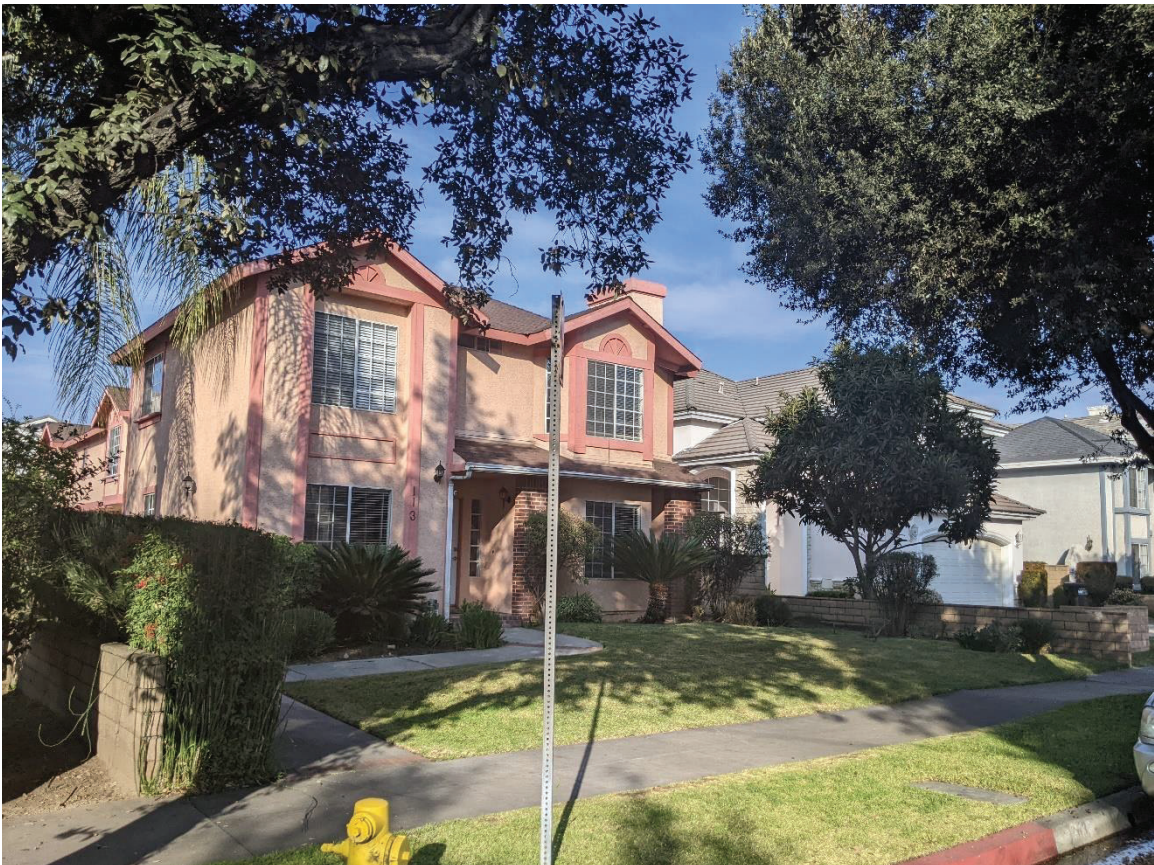
Figure 12 Adjacent property to the rear of the Arcadia Woman's Club: 113 Diamond Street.
