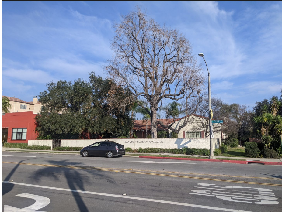
Arcadia Woman's Club building, eastern façade as seen from S. 1 st Avenue.
