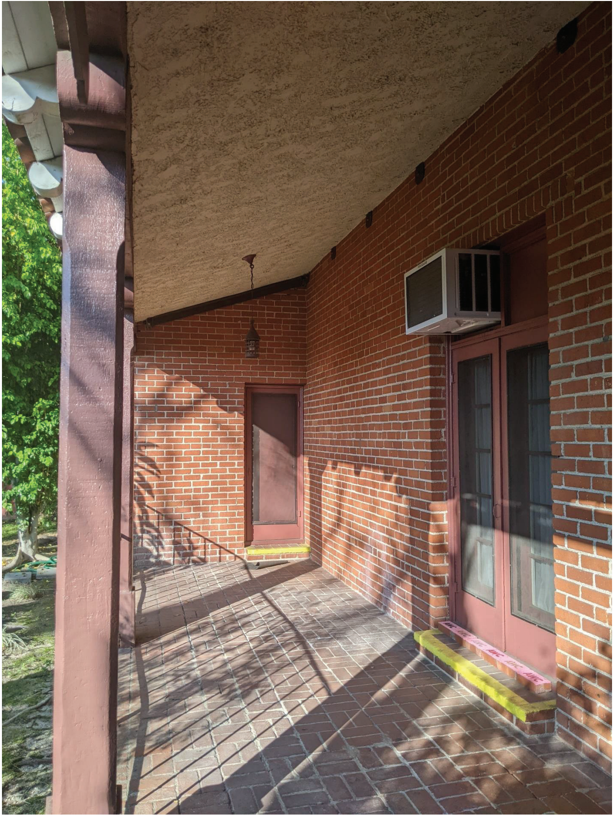
Figure 16 Under the covered porch looking north.
