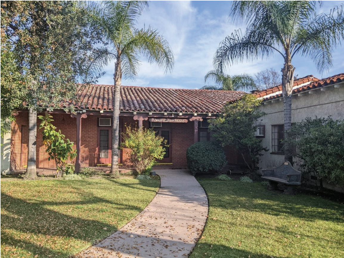
Figure 15 Front facade of the Arcadia Woman's Club showing the covered porch.
