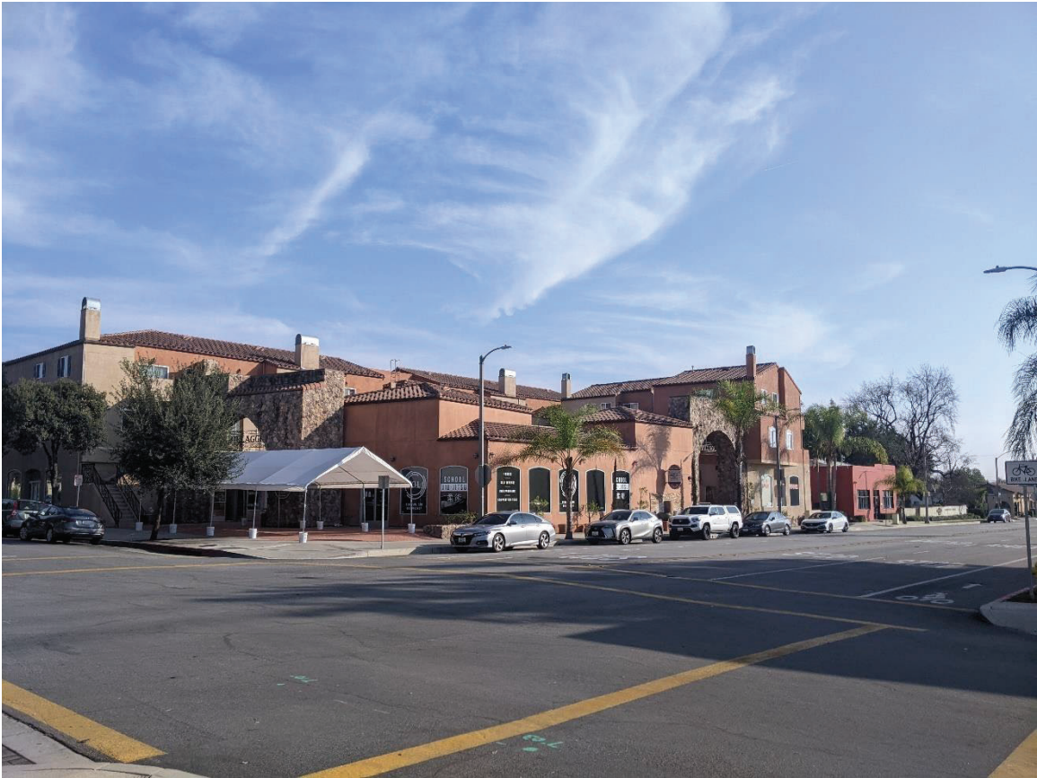
Figure 1 Looking toward the southeast corner of California Street and S1st Ave
