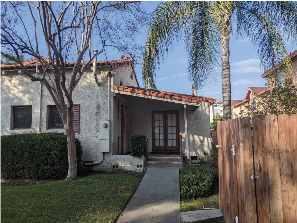
Figure 10 Looking north at the rear of the Arcadia Woman's Club building.
