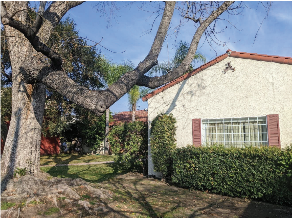
Figure 14 Front facade of the Arcadia Woman's Club building showing the vinyl window replacement.
