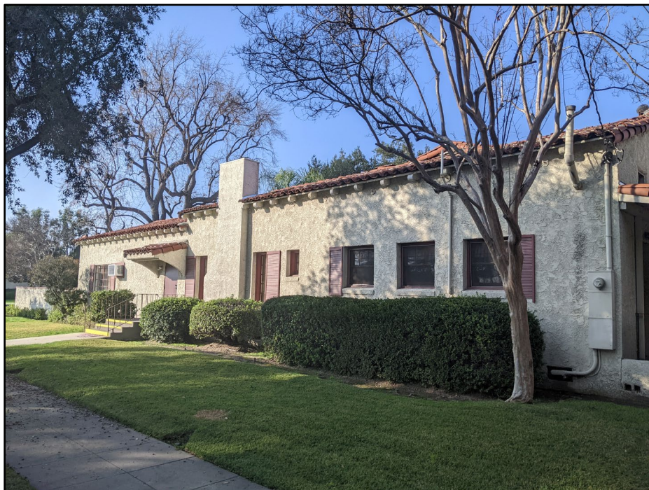
Southern façade of the Arcadia Woman's Club building as seen from Diamond Street.
