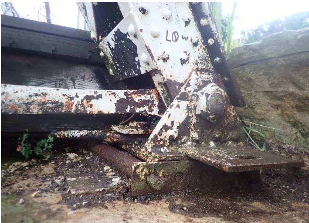
PHOTO 38 SOUTH ABUTMENT – WEST ROLLER BEARING
