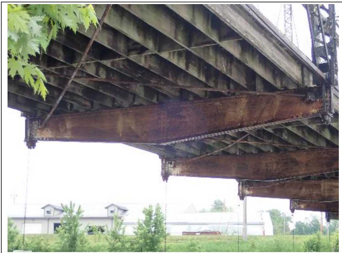
PHOTO 07 TYPICAL FLOOR SYSTEM (PANELS 9-10), LOOKING SOUTHEAST
