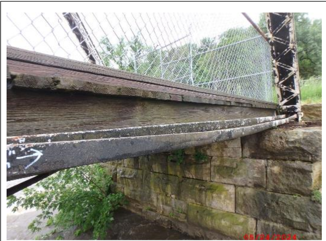
PHOTO 17 PANEL 1 – TRUSS, WEST BOTTOM CHORD EYEBARS
