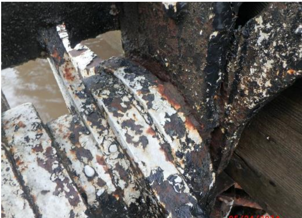
PHOTO 22 L4W – TRUSS, EYEBAR / PIN ASSEMBLY
