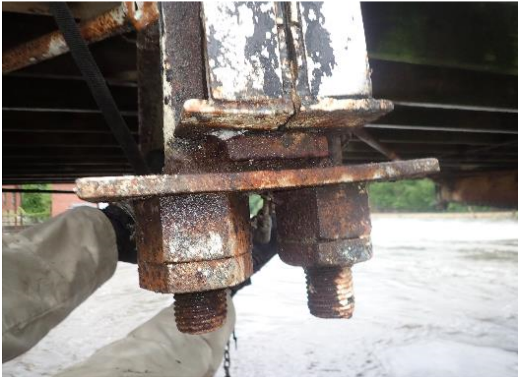
PHOTO 31 L8W – FLOORBEAM, WEST U-BOLT SPACER PLATE
