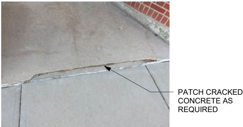
4 A190 CONCRETE RAMP REPAIR 1/4" = 1'-0"
