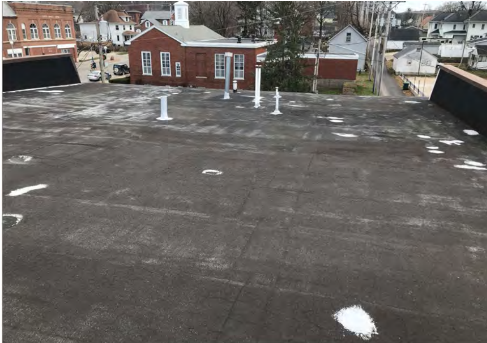
This photo shows the roof shared between buildings 209 and 211 W Main Street. The edge flashing and top layer roof membrane contain asbestos.
