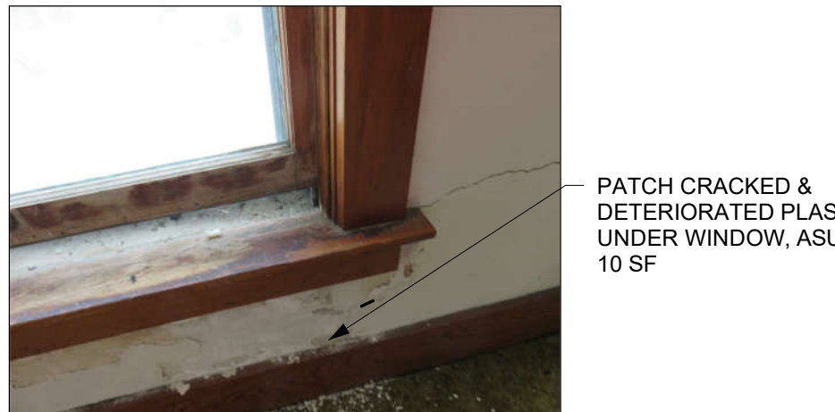
4 UPPER FLOOR INTERIOR WINDOW DETAIL A301 1 1/2" = 1'-0"
