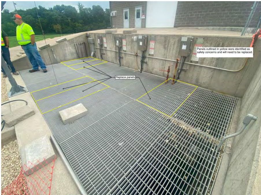
Figure 1: Panels to be replaced.
