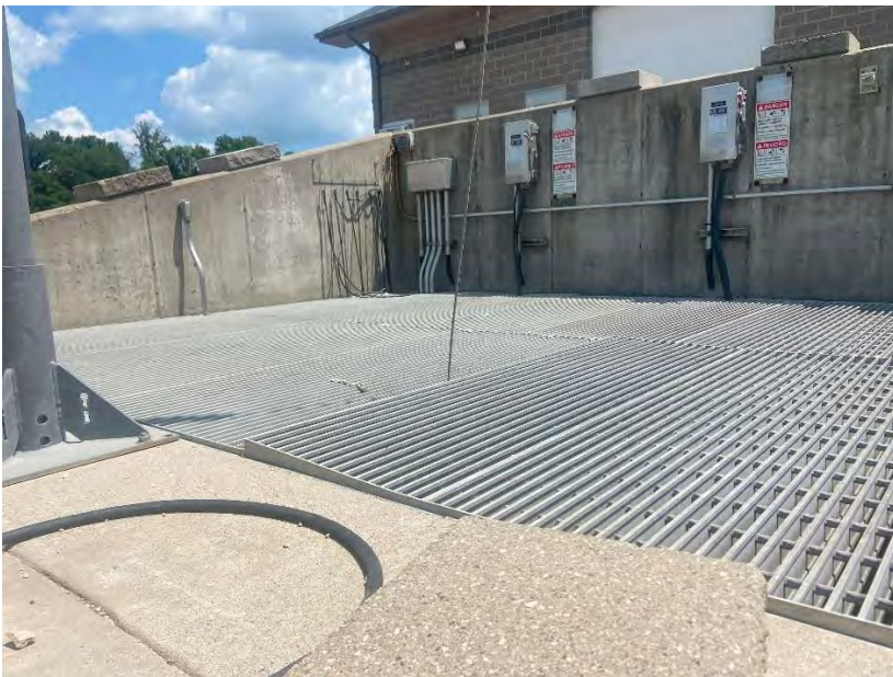
Figure 2: View of warped grating in front middle section.
