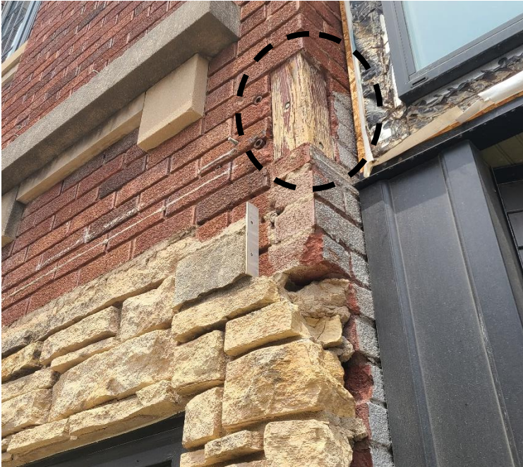
Photo 4 – Wood infill of brick on 106 E.
