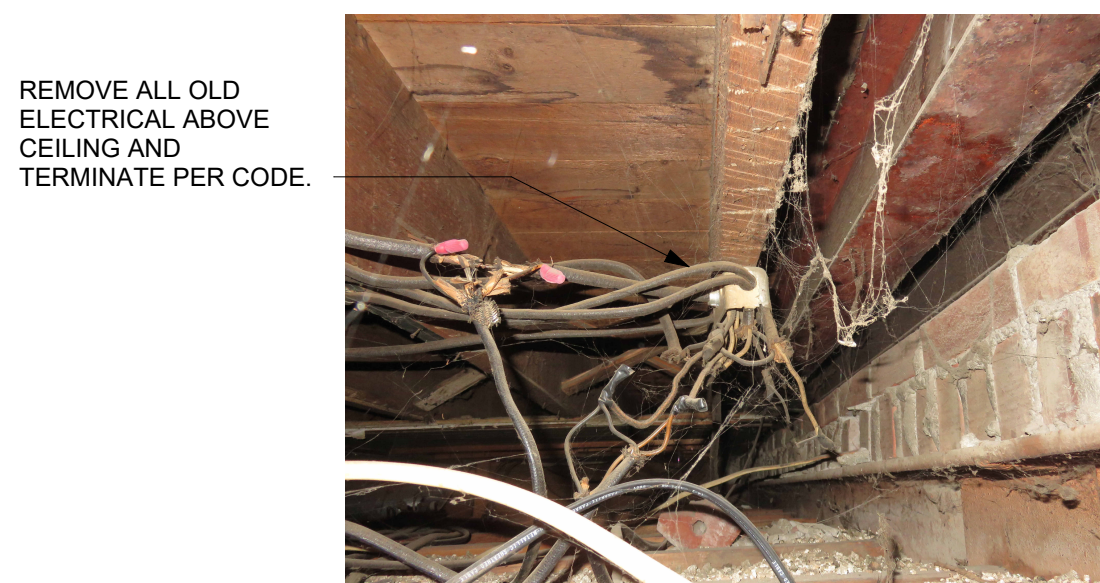
8 A112 EXIST. ELECTRICAL ABOVE CEILING 1/8" = 1'-0"
