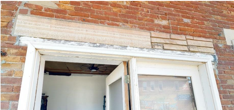
Photo 1 - Door 100E-3 wood and stone lintels.
