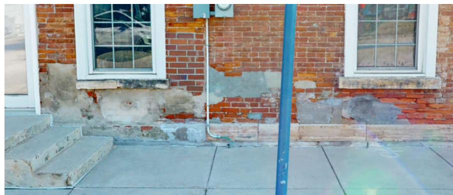
REMOVE PARGE FROM BRICK IN THIS AREA. REPLACE WITH BRICK TO MATCH.
