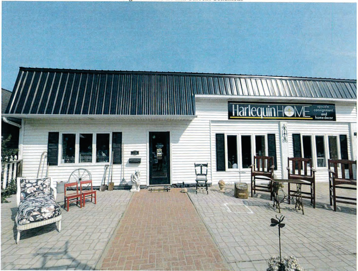
Figure 21: 216 E Main Current Conditions
