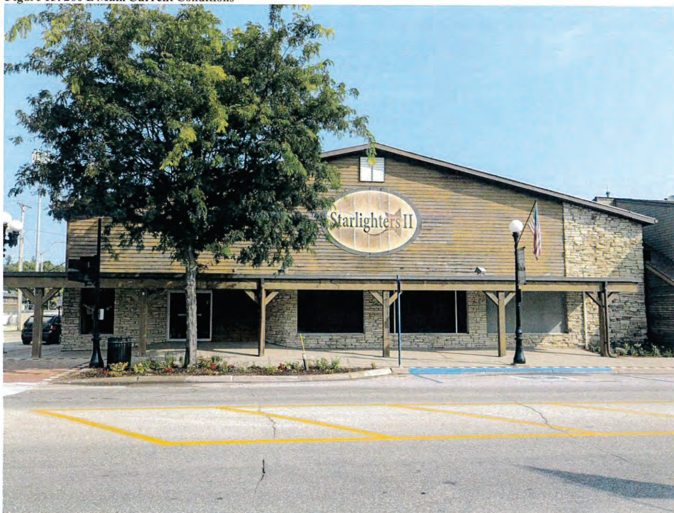
Figure 15: 200 E Main Current Conditions
