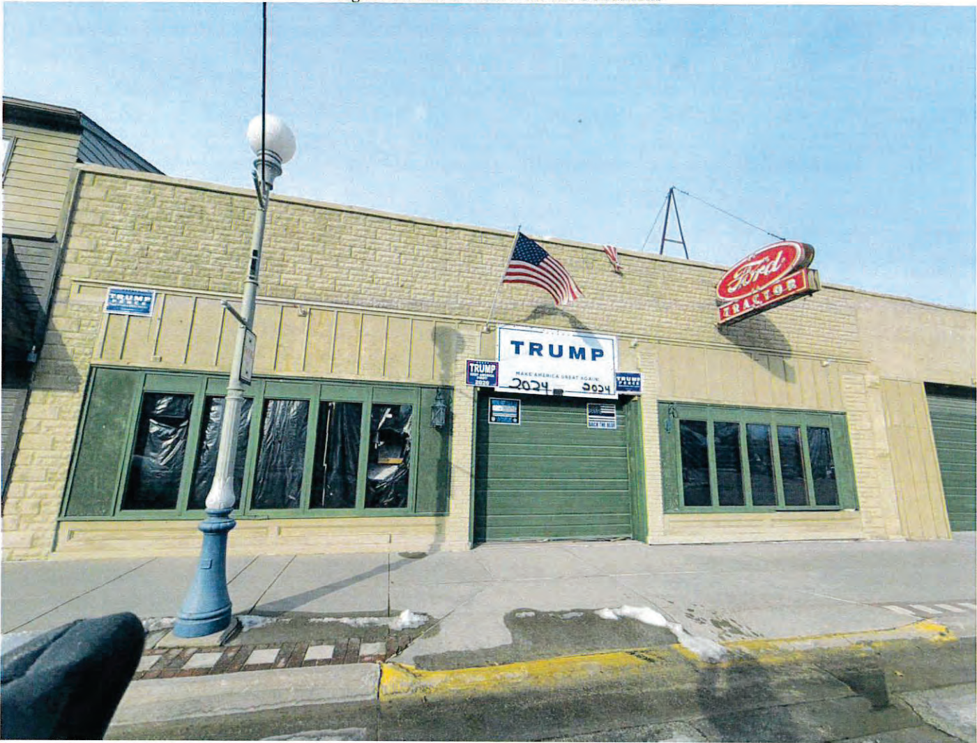
Figure 17: 210 E Main Current Conditions
