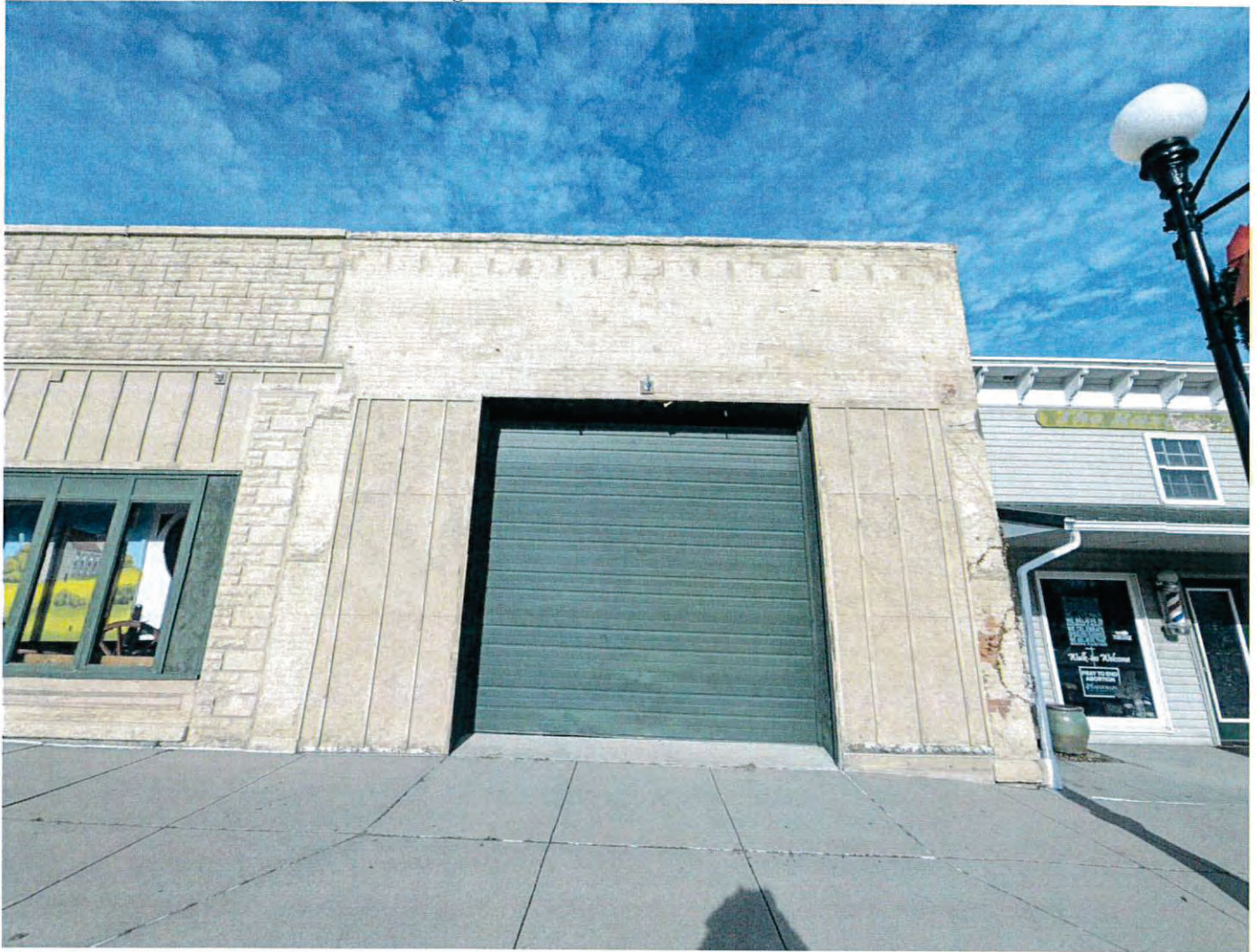
Figure 19: 212 E Main Current Conditions
