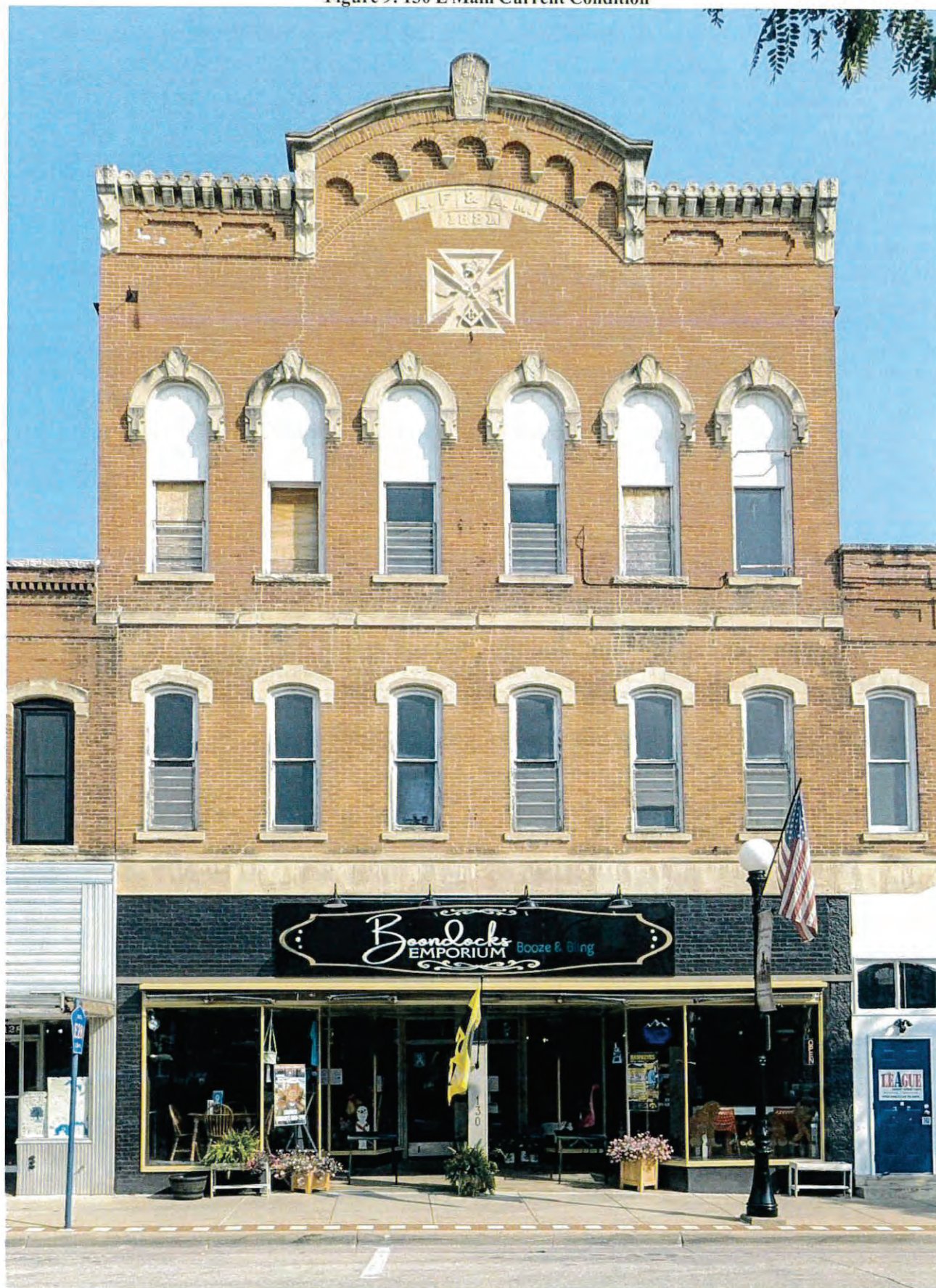
Figure 9: 130 E Main Current Condition
