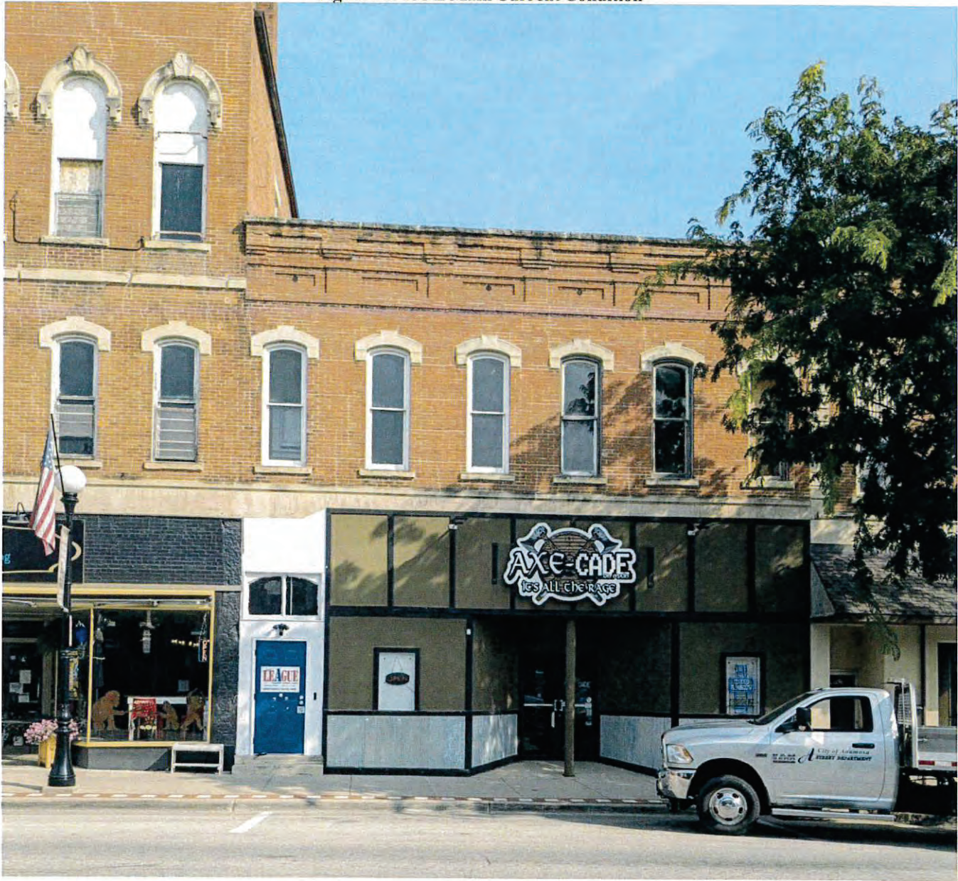
Figure 11: 138 E Main Current Condition
