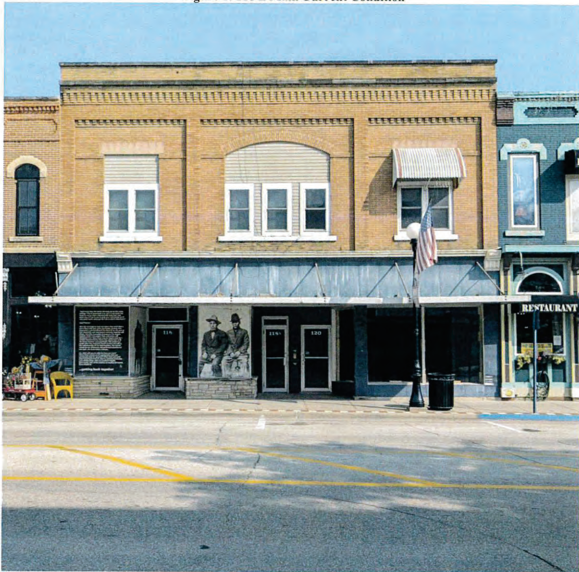
Figure 1: 118 E Main Current Condition
