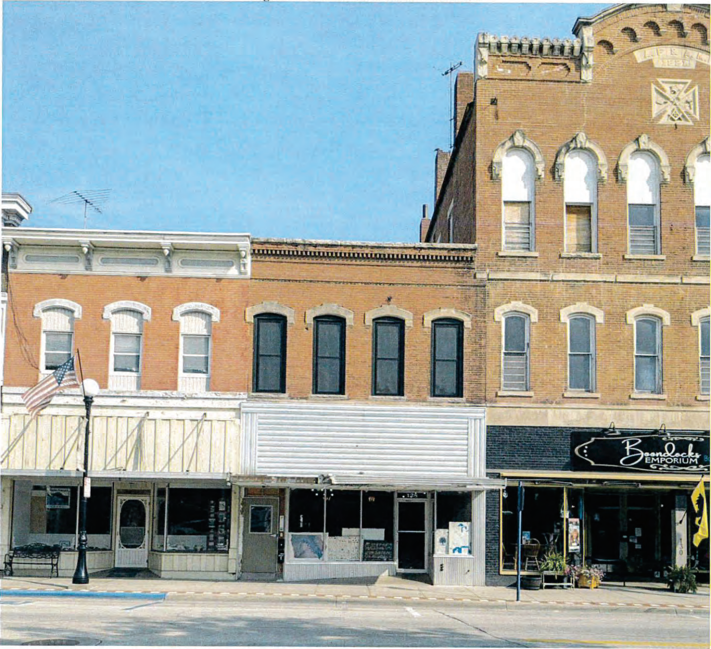
Figure 7: 128 E Main Current Condition
