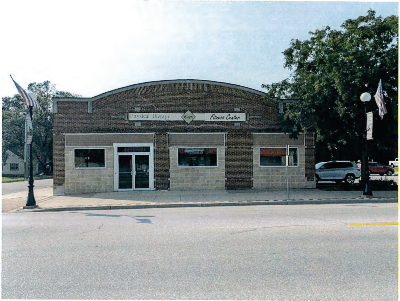
Figure 23: 315 E Main Current Conditions
