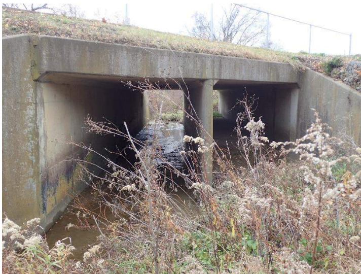
Photo 3 – Side View Looking South
