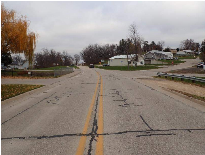
Photo 1 – Road View Looking East
