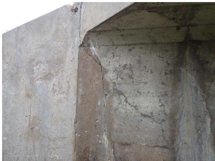
Photo 8 | West Outlet Wingwall
