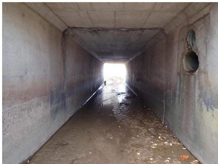
Photo 5 – East Barrel Looking North
