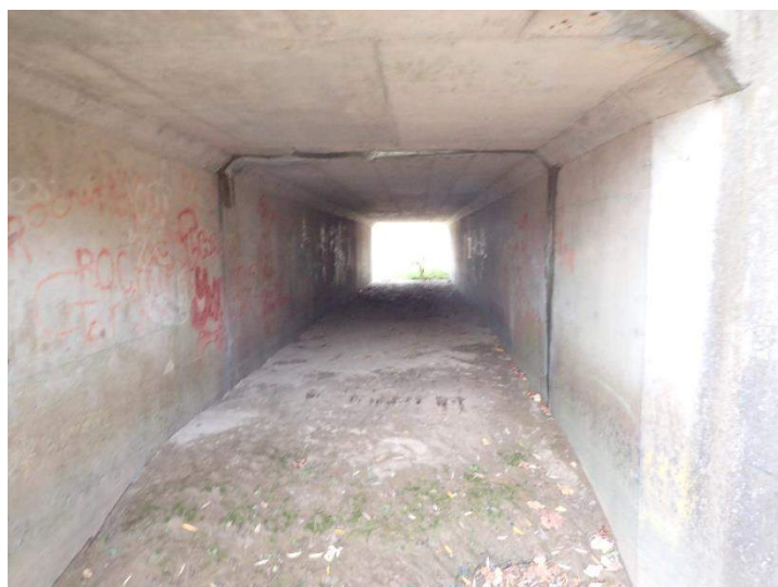
Photo 6 – West Barrel Looking South
