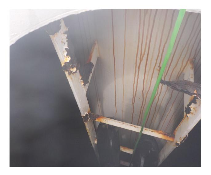
Recommendations: Interior ladder needs to be removed and replaced with a new OSHA approved ladder and fall protection cable installed to new ladder.
