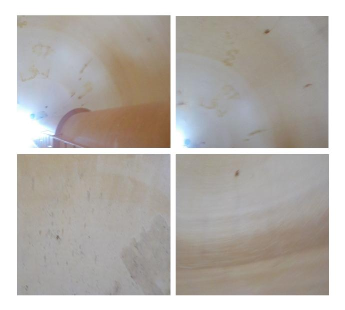
Recommendations: It's time for the community to start the budgeting process to have the interior liner abrasive blasted to a near white finish (SP SSPC-10) and a new 2 coat epoxy liner installed. This process should be done in the next 1-2 years
