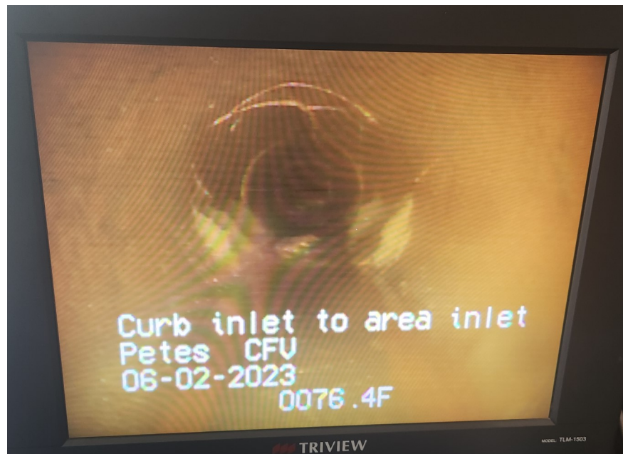
Cracked Sewer Pipe
